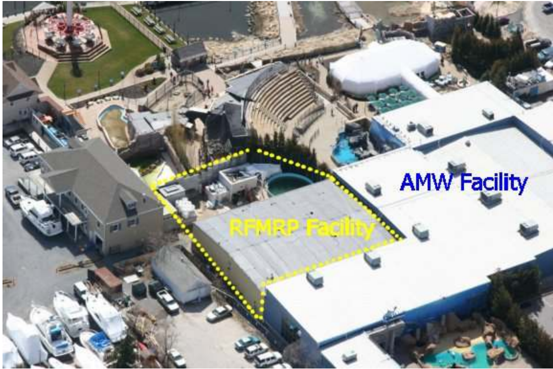
Figure 2.0. RFMRP facility located at Atlantis Marine World Aquarium
